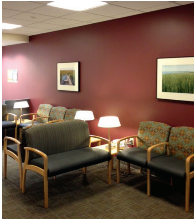
Dover Family Practice Qt PRO 600 Sound Masking Installation
